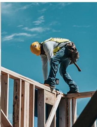
Factory & Construction site
